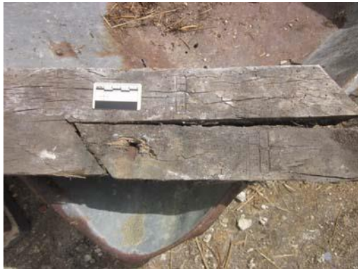
Figure 4 Wall-plate scarf joint II
