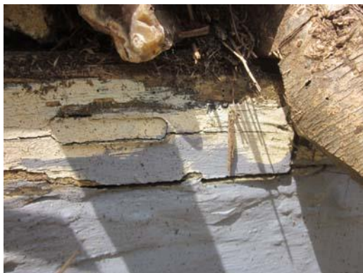
Figure 6 Shadow crossing end of loose tenon
