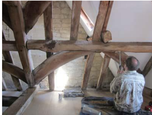
Figure 9 Dan Miles drilling a roof timber
