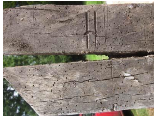
Figure 5 Assembly mark and setting-out lines
