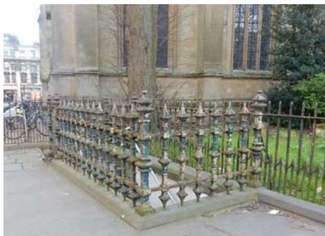
Figure 4 East toilet entrance (Lucy design)
