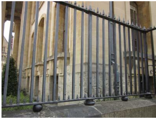
Figure 8 Clarendon building railings
