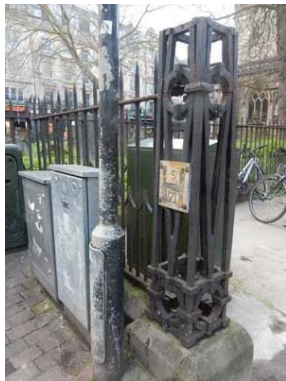
Figure 5 Cast iron pillar
