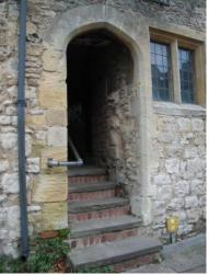
The pedestrian access from Thames Street to the Abbey precincts has been roughly cut out of the Chequer building at some stage. A brick partition wall has been inserted to form an alley way or slype (Fig.15)
