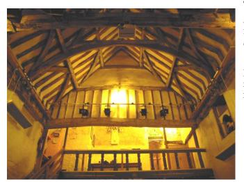
There are few pegs visible from ground level, it is likely that the roof was pegged from the outside.
