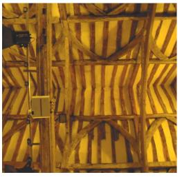
By the 19<sup>th</sup> century the Checker Hall had domestic accommodation on three levels. The tie-beams have evidence for joists running east-west to support an attic floor, and there was a first floor inserted within the main hall structure, partly supported by the central stack. As far as internal partitions are concerned, the central tie beam has mortices for studs in the soffit of its southern half, and the western truss has evidence of mortices in the collar soffit.
