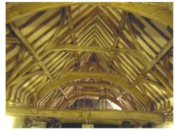
intermediate trusses also with high collars but without the braces or tie-beams Between the trusses are two tiers of buttpurlins, each braced to the principal rafters by curved windbraces.
