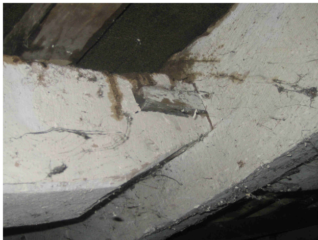
Figure 14 Free tenon in rear wing roof
