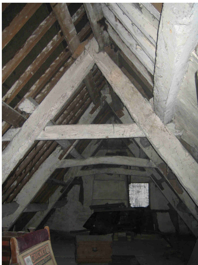
Figure 13 Roof of rear range looking north
