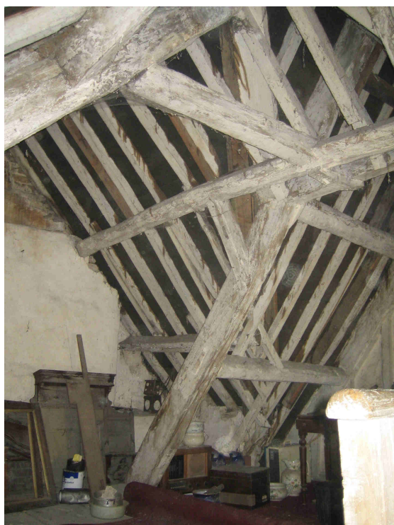
Figure 11 To the left is the west gable of the front range. In the centre one of the trusses of the rear wing extends into the roof of the front range.
