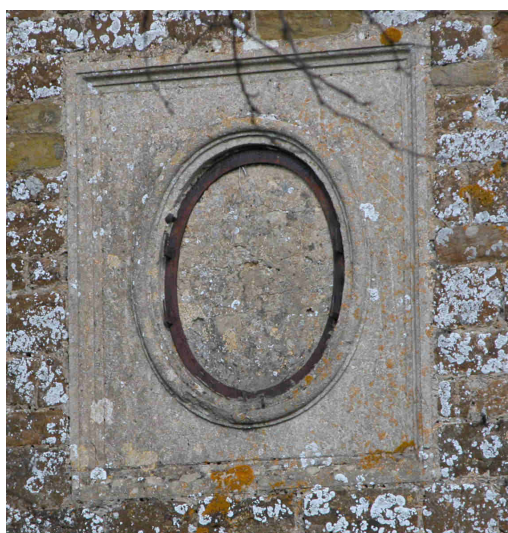
Figure 4 Former elliptical window
