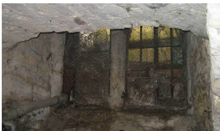
Figure 12 Stone mullion window to cellar
