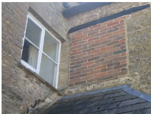
Figure 10 Blocked window at join of C and D
