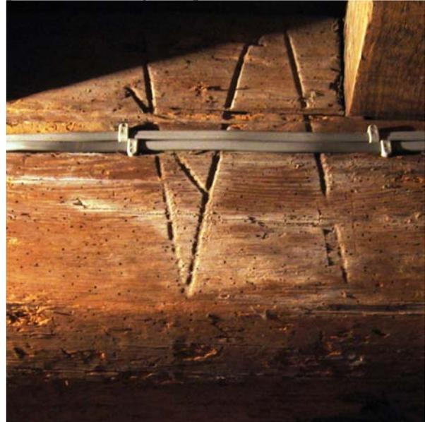
Above: an example of Baltic timber marks recorded by OBR members in Abingdon Long Gallery. This set is on a softwood transverse beam inserted as an 18<sup>th</sup> century alteration to the ground floor.
