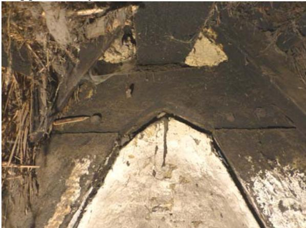
This recent discovery at Sutton is the saddle at the apex of an open cruck frame, in the centre of a 2-bay open hall. It is heavily smoke blackened, as is the thatch around it, particularly to the right, although the truss has later been infilled with wattle and daub, and limewash added over the soot encrustation. It is exciting to encounter 'new' old roofs as unexpected survivals, especially to know that the blackened water reed base coat and hay roll of the thatch above the substantial ridge
