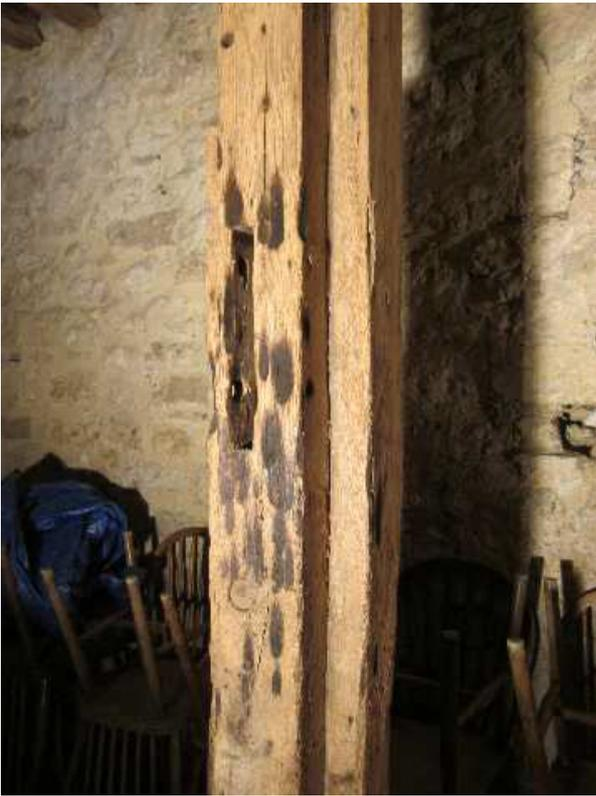
Above: another example of timber marks recorded by OBR members in the 15<sup>th</sup> century Abingdon Long Gallery. Burn marks on a timber post of the ground floor. Note that they have been made after the horizontal rail was removed (empty mortise) indicating that they post-date the original structure.
