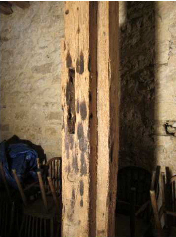
Above: another example of timber marks recorded by OBR members in the 15 th century Abingdon Long Gallery. Burn marks on a timber post of the ground floor. Note that they have been made after the horizontal rail was removed (empty mortise) indicating that they post-date the original structure.
