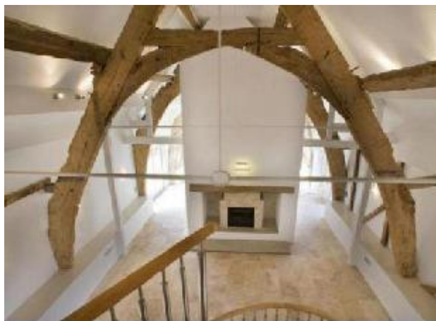
Above: the 14 th C cruck barn at Rectory Farm, Northmoor, W.Oxon, before and after conversion to a cosy home. Photos: left David Clark, right from estate agent's particulars.
