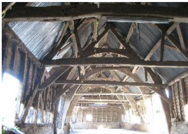
Above: the 14 th C cruck barn at Rectory Farm, Northmoor, W.Oxon, before and after conversion to a cosy home. Photos: left David Clark, right from estate agent's particulars.
