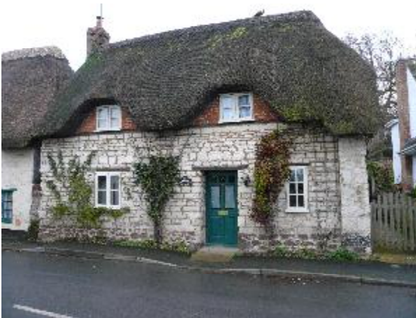
17 th C cottage built of chalk on sarsen base (and attic walls raised in brick).
