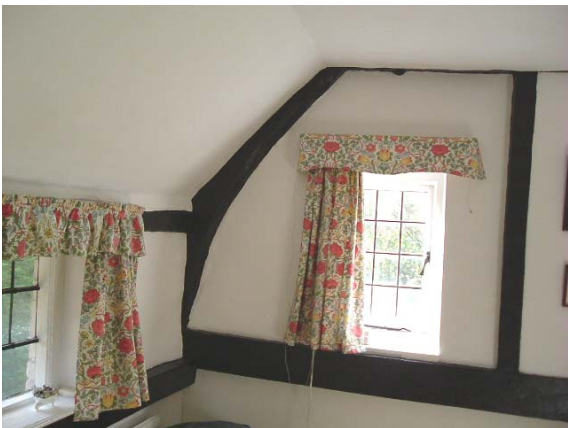
Base cruck used to raise eaves height
