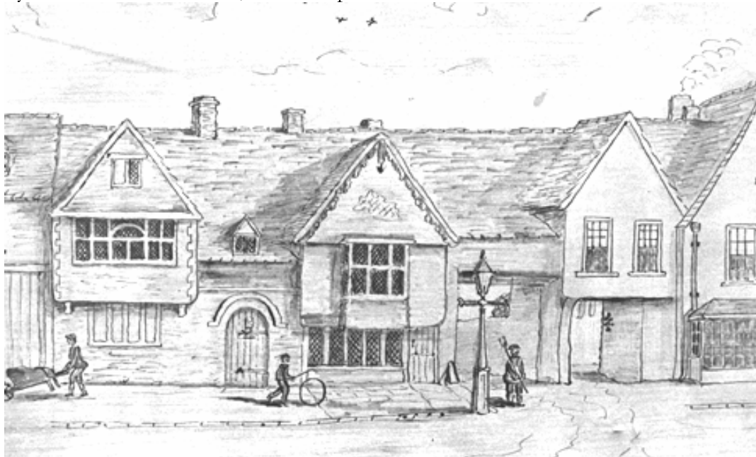
Demolished house facing Market Square
