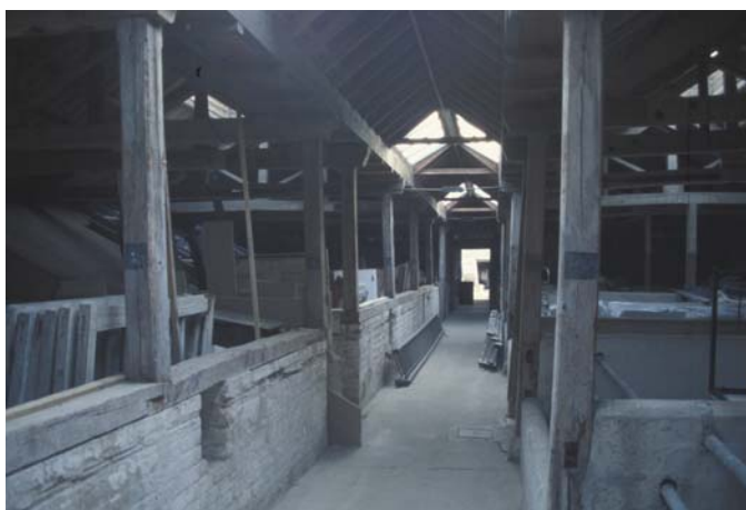
Cattle fattening stalls at Coleshill with central passageway for a tramway
