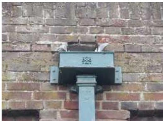
**Figure 5** Rainwater goods rear detail
