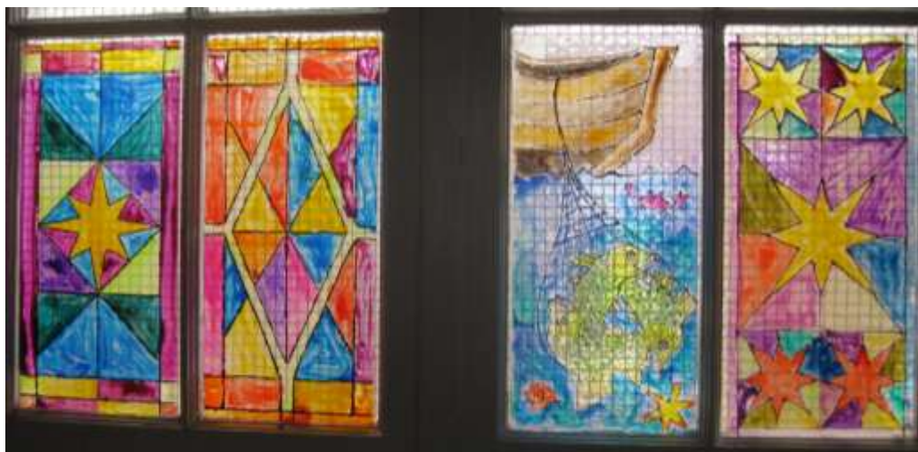
Window 3 East wall 3
