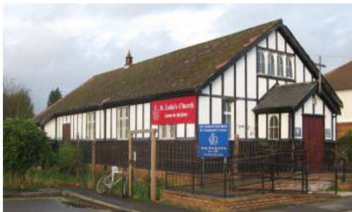
Figure 1 St Luke's, Canning Crescent
