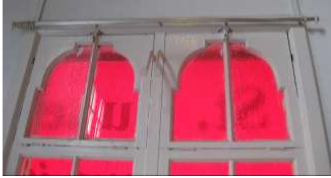
Figure 8 Detail of windows
